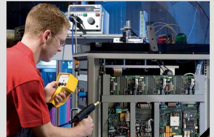
EN60204 test at a service cabinet
